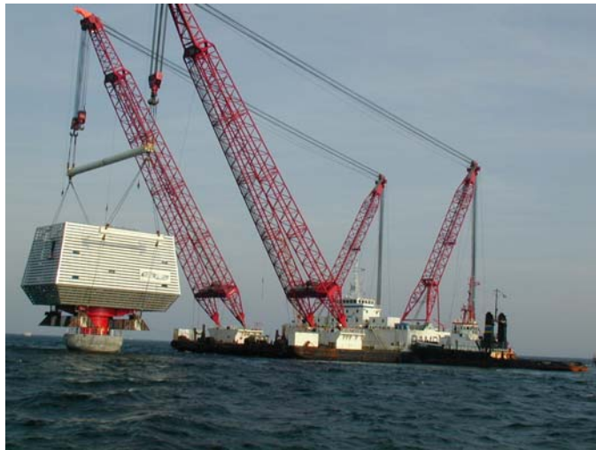
Fig. 13 Installation of Entire Topside
