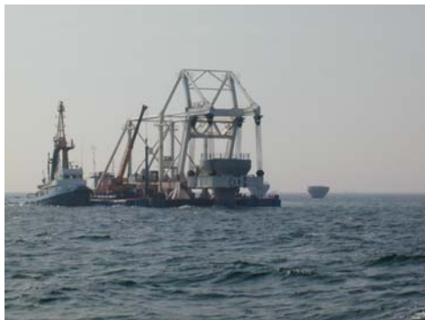
Fig. 7 Installation of Foundation.
