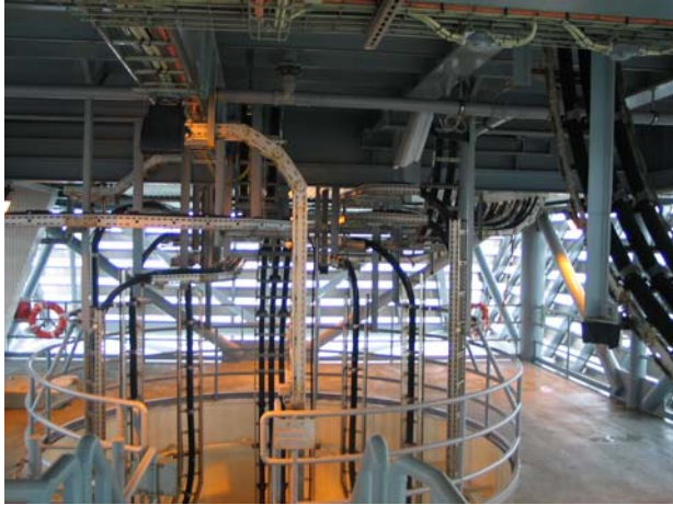
Fig. 5 View of Cable Deck.
