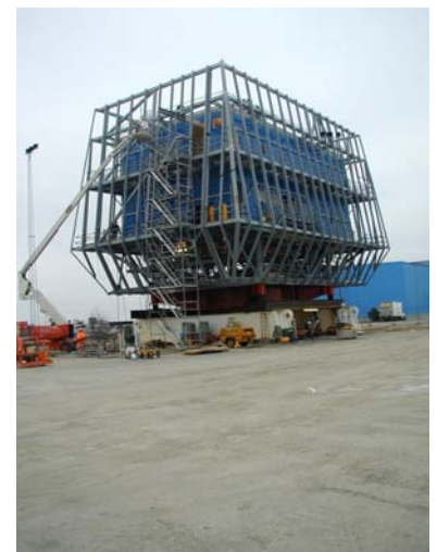
Fig. 12 Topside during Fabrication in Yard.
